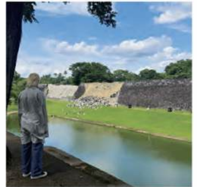
地震で崩れた熊本城の石垣を見つめる井上文太氏 Bunta Inoue looking at the earthquake-damaged stone walls of Kumamoto Castle.
